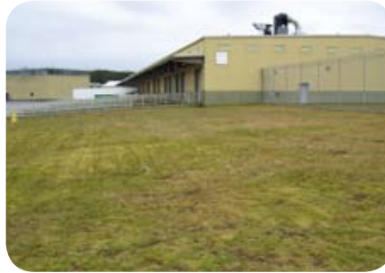
Future site for new furniture factory building located at SCCC.
